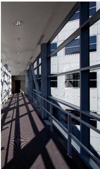
Figure 8.2: Fixed windows in corridor
