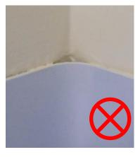
Figure 30: Gap between skirting and walls
