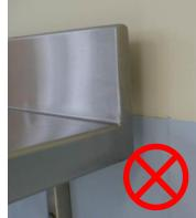
Figure 29: Gap between bench fitting and wall
